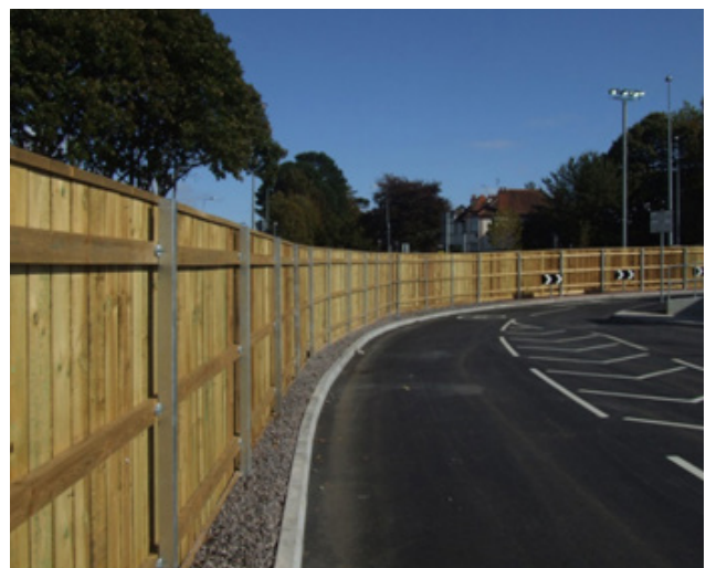
Figure 14: Roadside noise barrier fencing Photo: AlphaFence
