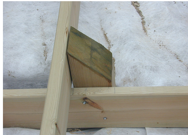
Figure 15: Top of post sloped to shed water
