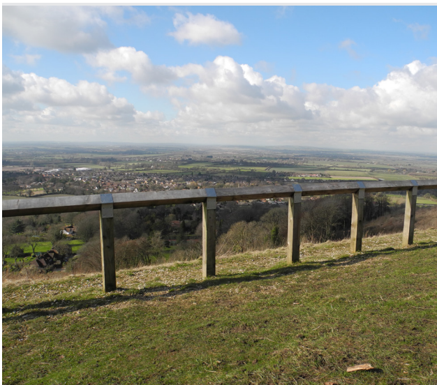
Figure 2: Hilltop safety fencing
